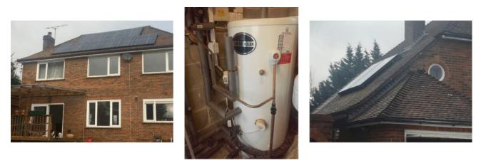
Figure 2: Example of one grant recipient. Left: A ten panel 4kW solar photovoltaic system. Centre: The new solar hot water tank, to store the solar generated hot water. **Right**: A double panel, flat plate solar thermal collector. Renewables were complemented by cavity wall and loft insulation.
