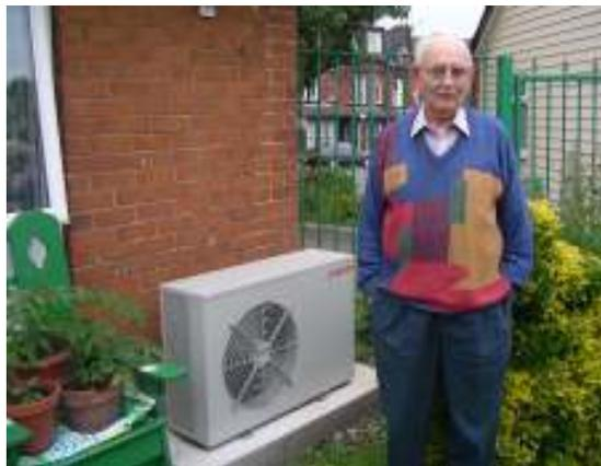
ASHP components have a design life of approximately 20 years compared to high efficiency gas boilers which have a 7/10 year life. With a gas boiler costing in the region of £700 and an ASHP costing around £2200, the whole life costs are very similar.
