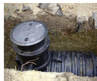
Rainwater tank being submerged at Oak Tree House
