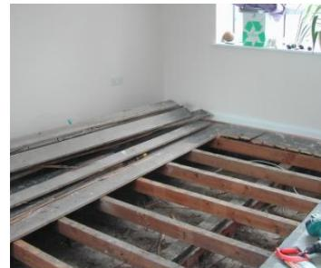
After the insulation has been laid the floor boards can be replaced and any gaps should be blocked with regular tube sealant such as silicon to prevent any draughts coming up through floor. The edge of the carpet or flooring should also be sealed around the skirting board.
