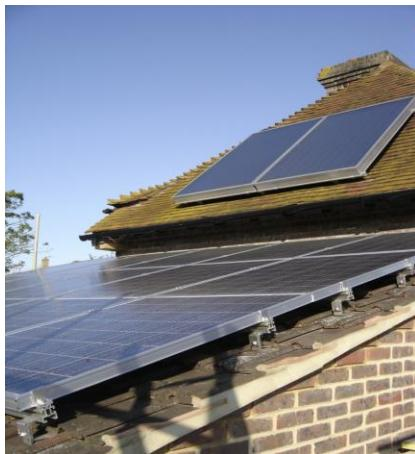
Hybrid technology solar cells use a combination of monocrystalline and amorphous solar cells which can provide a higher efficiency than single monocrystalline cells and therefore require less roof space. They are however, more expensive.
